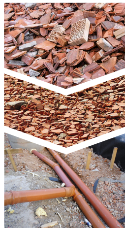
Refilling pipelines 0/64
