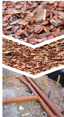
Refilling pipelines 0/64
